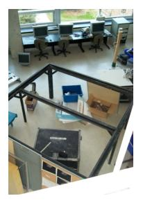
(b) View of the floor support taken from the 2<sup>nd</sup> story of the VGR lab. A catwalk around the space provides access to the projectors and mirrors. Note that IVY's floor is located 4' above the physical floor of the lab.
